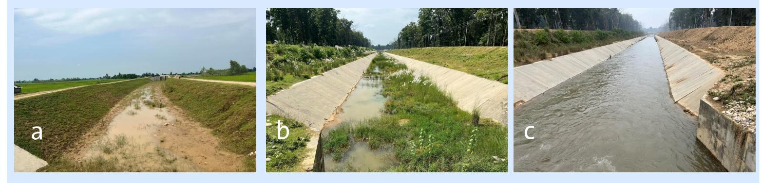
Fig.1. (a) earthen canal with low conveyance effieciency with high seepage and percolation loss , (b) concrete lined canal but not well maintained with low effieciency, (c) high effieciency well maintained canal lined with concrete.
