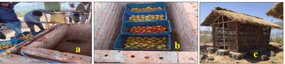
Fig. 6: Completed (a,b) tomato zero energy bricks evaporative cooler and (c) potato ventilated storage structure in Arsi zone in 2022
