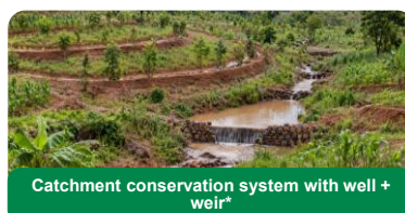
Catchment conservation system with well + weir*
