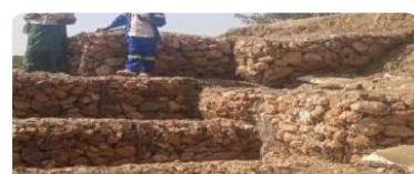
Stone water-harvesting structure
