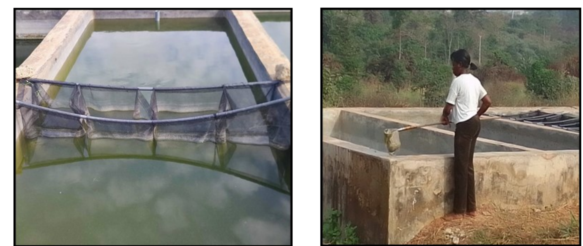
Fig. 2: Concrete tanks and Hapas set up
