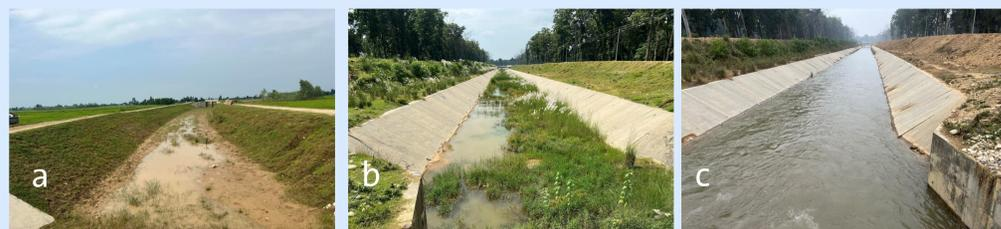
Fig.1. (a) earthen canal with low conveyance efficiency with high seepage and percolation loss, (b) concrete lined canal but not well maintained with low efficiency, (c) high efficiency well maintained canal lined with concrete.
