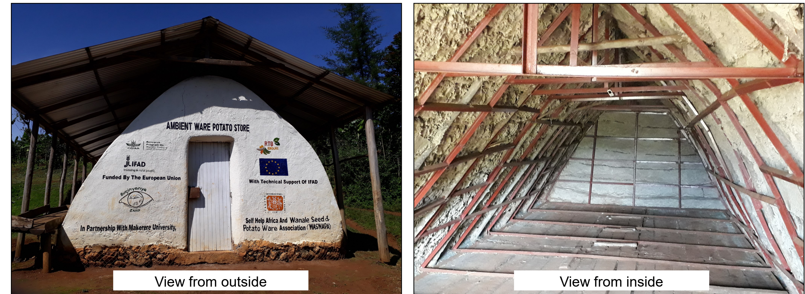
Figure 2: Improved group ambient ware potato stores piloted in Uganda (50 t storage capacity, 10 years lifespan, unit cost of approximately USD 15,000).
