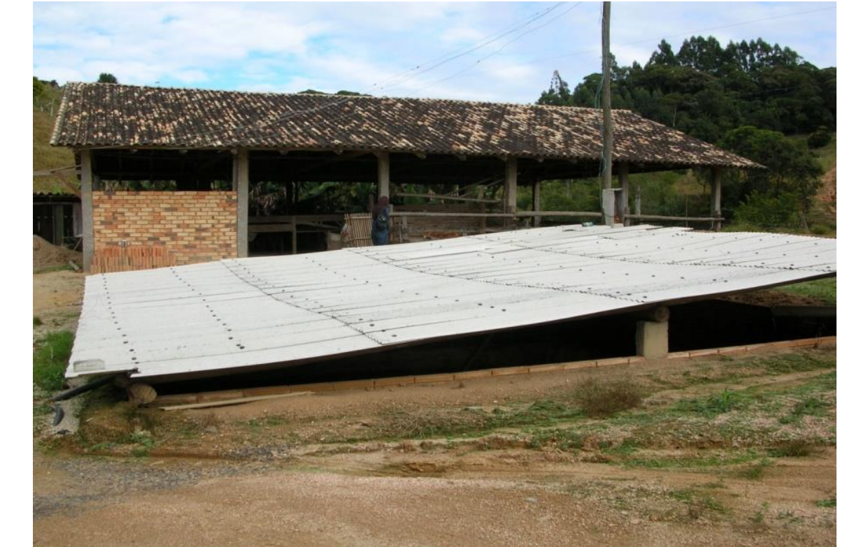
Figure 2. Storage tank (residues)
