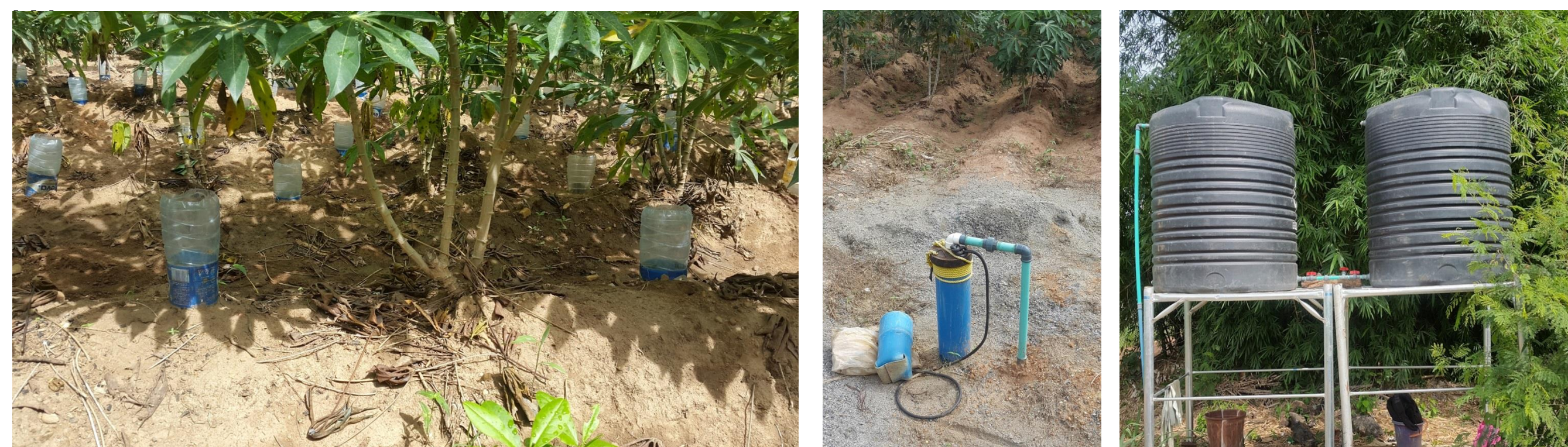
Figure 1: Used bottles inserted upside down into the soil to supply water with minimum losses (left), bore hole to pump water (middle), storage tanks (right).
