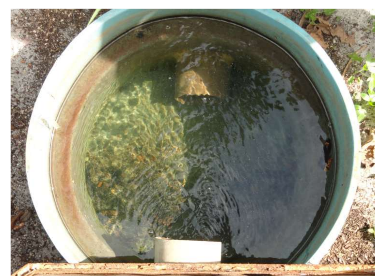
Fig. 9 Result: Clear water, ready to be used for agronomic fertigation.
