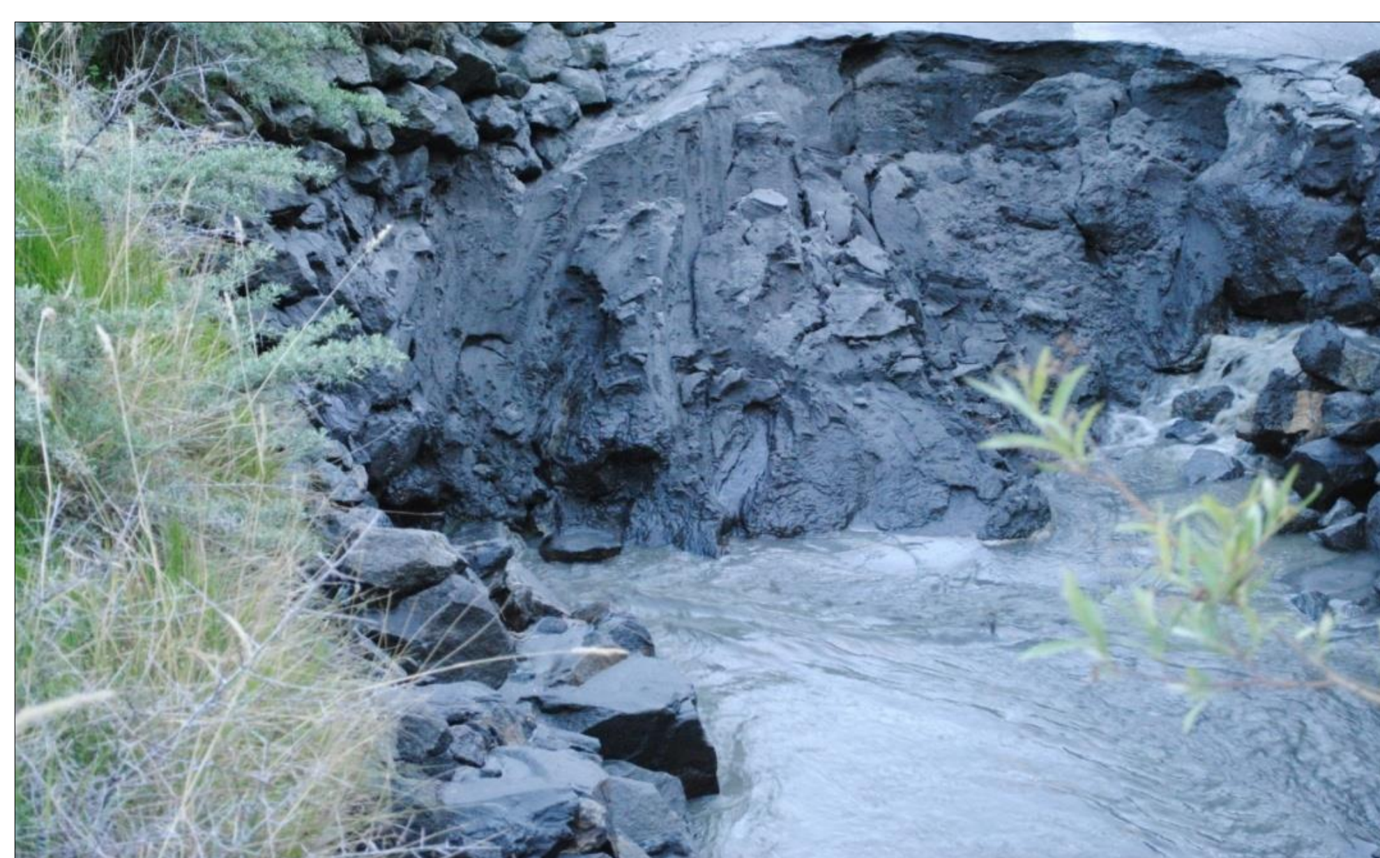
Fig. 2: Traditional sedimentation tank at which channel sediments are discarded and flushed away by river or creek waters.
