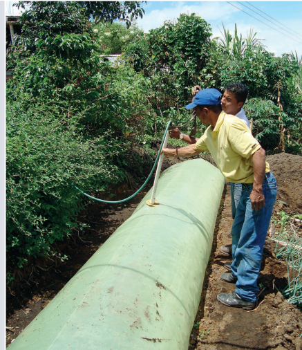
Photo 1: Biodigester installation by a member and promoter of ASPROINCA
