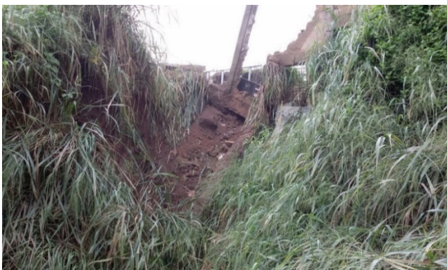
Figure 2: wastewater discharge from CU
