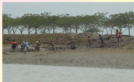
Fig. 4 Local people repairing dam collectively*
