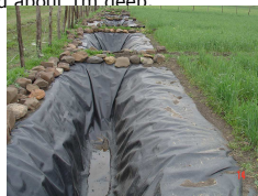
Fig. 6. Runoff collection ditches
