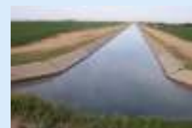
P 2. Public river irrigation system
