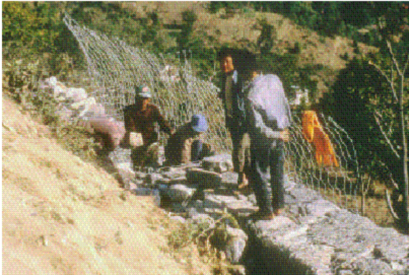
Check dam-Gabion
